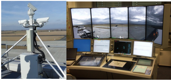
Fig. 1. Remote tower installation with 200°-panorama and pan-tilt zoom camera sensor system at the tower roof (left photo), and operators workplace with 40"-HD-format displays (right)
