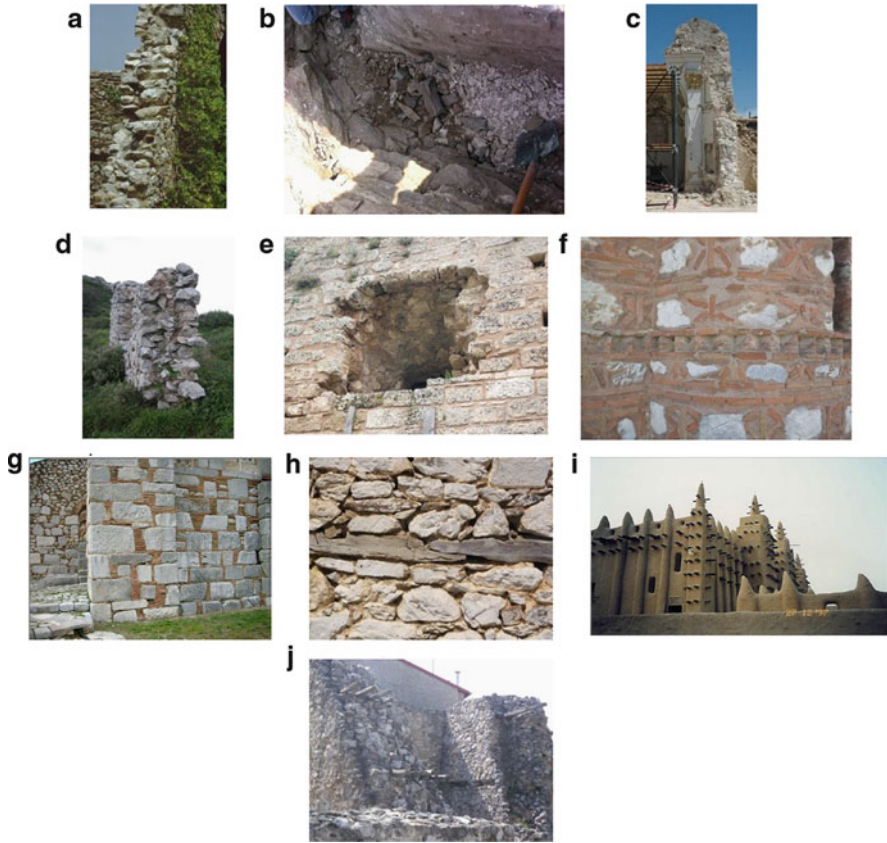
Fig. 8.1 Examples of types of historic masonries. (a) Double-leaf stone masonry with sporadic header stones. (b) Three-leaf stone masonry - thick interior leaf with very large voids. (c) Poor quality three-leaf rubble stone masonry. (d) Three-leaf rubble stone masonry. (e) Multi-leaf masonry with high mortar volume. (f) Mixed stone-brick masonry with large mortar volume. (g) Mixed brick-stone masonry of good quality. (h) Timber reinforced rubble stone masonry. (i) Timber reinforced adobe. (j) Timber reinforced multiple leaf masonry
