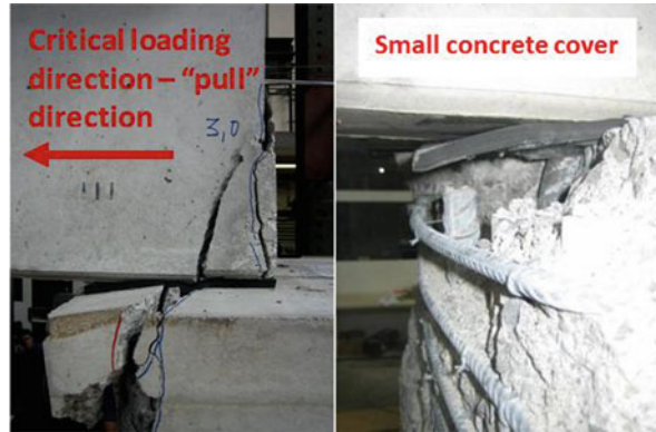
Fig. 4.34 Failure in the case of small concrete cover and in the case of the insufficient tension strength of concrete and stirrups surrounding the dowel
