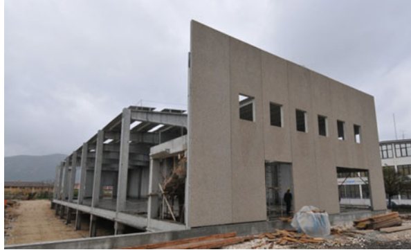
Fig. 4.7 Structural system of most precast industrial buildings designed for seismic action remained undamaged during recent Italian earthquakes
