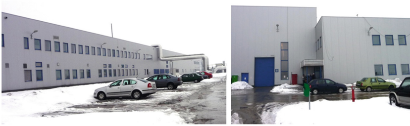
Fig. 4. Photos with case study building (difference in height between production unit and warehouse is visible in the right photo).
