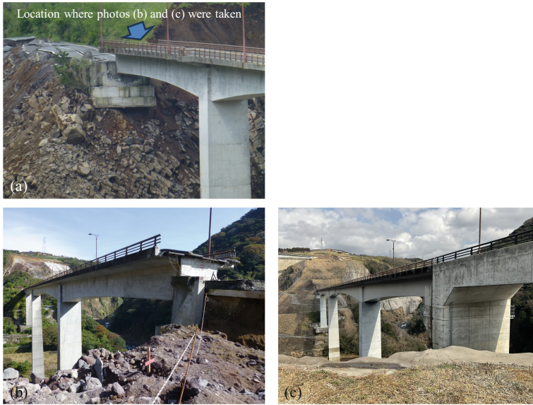
Fig. 8. Example of robust structures against catastrophic hazards (a) and (b) taken after the 2016 Kumamoto earthquake; and (c) taken after the reconstruction of the abutment. Note that all pictures were taken by the second author.
