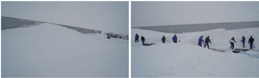
Fig. 6. Snow accumulated at the contact between the two buildings.
