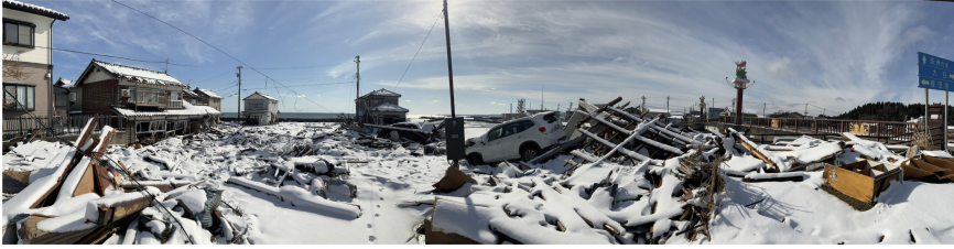
Fig. 6. Tsunami damage in Suzu City and disaster waste generated by the 2024 Noto-Hanto earthquake. Note that the picture was taken by the second author.
