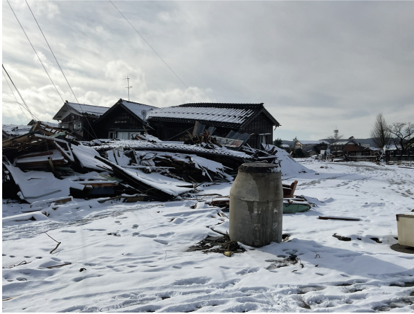
Fig. 4. Collapse of classical wooden Japanese houses due to ground motion, tsunami and/or liquefaction caused by the 2024 Noto-Hanto earthquake. Note that the picture was taken by the second author.
