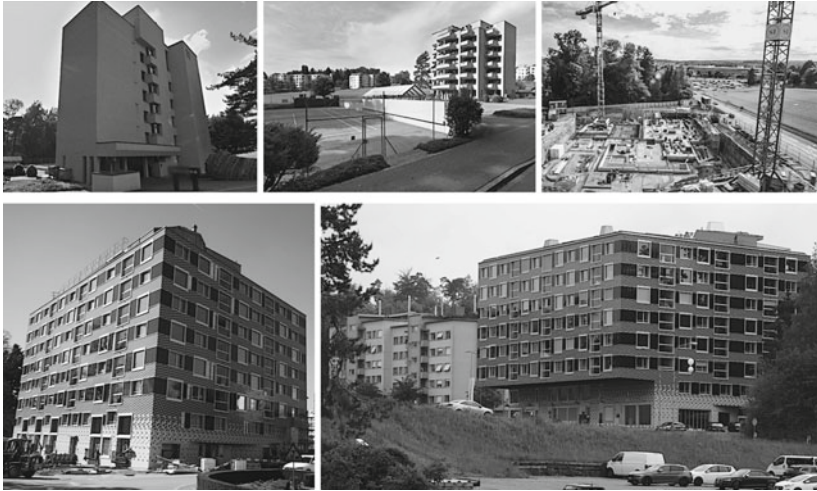
Fig. 4.11 Photographs of Klotten Southern district settlement before (top) and after (below) demolition and total replacement construction and densification ( Sources Google Streetview; own photographs)
