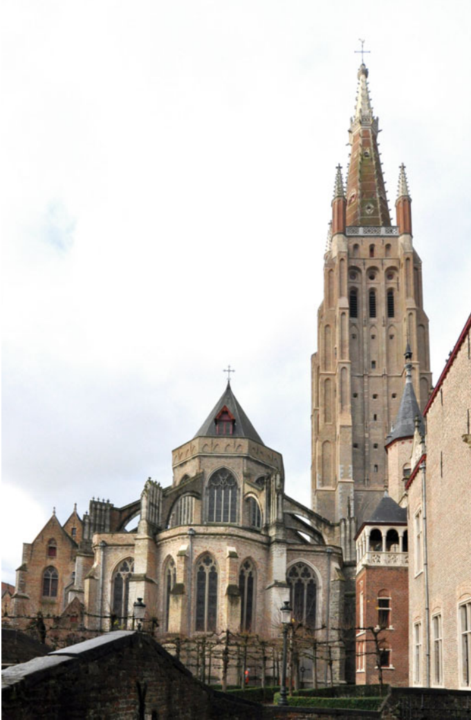
Fig. 4 Bruges, choir and tower of Our Lady, the tower was begun around 1290 and the trunk was finished in the third quarter of the fourteenth century. The spire was built in the first half of the fifteenth century, but the current spire dates from the nineteenth century (Hurx)
