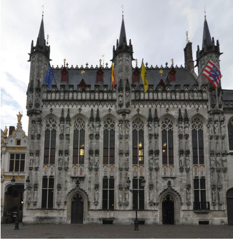
Fig. 12 Bruges, town hall, 1376–1421 (Hurx)
