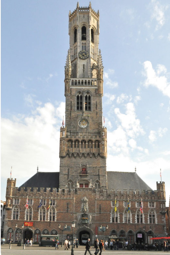
Fig. 5 Bruges, belfry of the cloth hall, begun in the last decades of the thirteenth century, second storey dates from the middle of the fourteenth century, and the octagonal lantern was added in the 1480s (Hurx)
