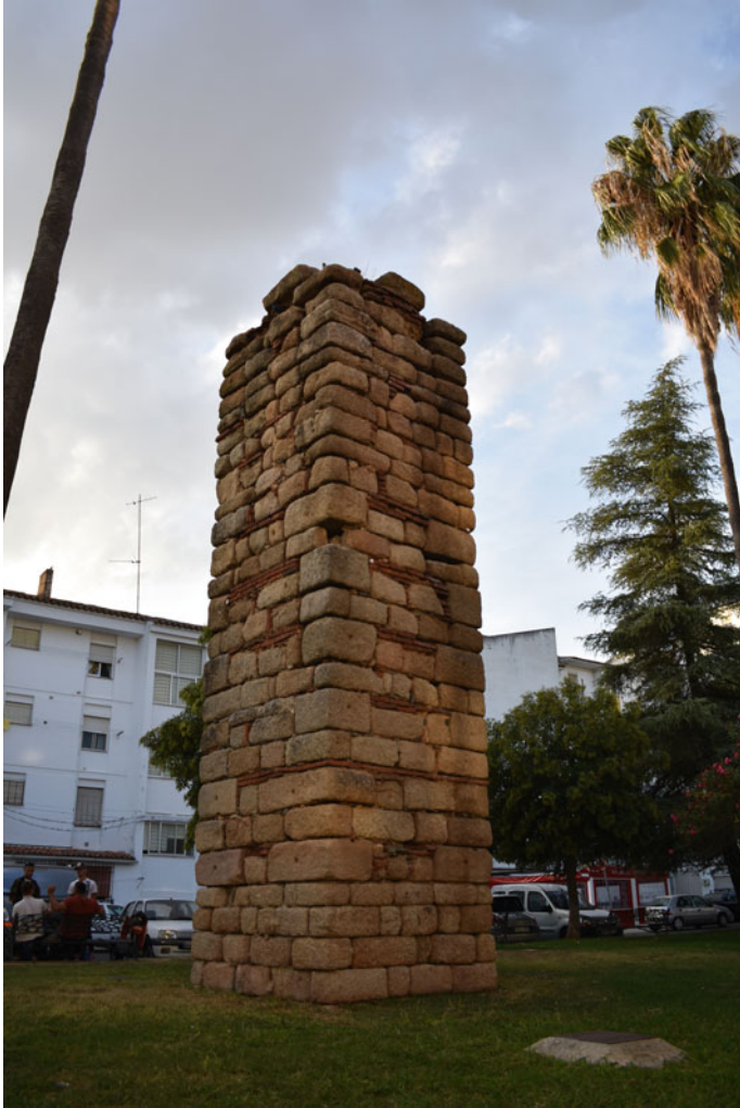
Fig. 2 Failed sixth-century repair of a pillar of the Los Milagros aqueduct, Mérida
