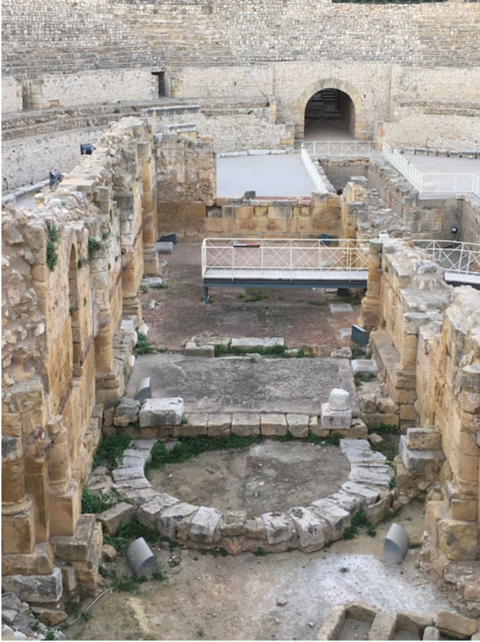
Fig. 6 Foundations of the sixth-century basilica (under standing walls of the later, medieval church) built in the Roman amphitheatre of Tarragona
