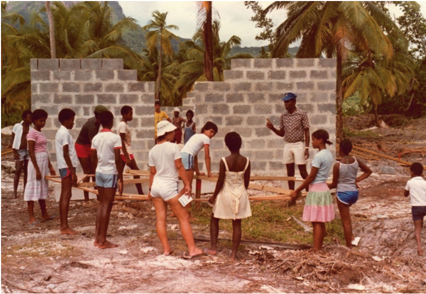
Image 27.3 A work crew of students and animateurs (youth leaders) prepare to raise a roof truss in a classroom. (Image: Hubert Murray, 1981)
