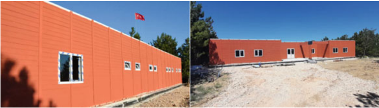
Fig. 14.11 1-story building field demonstration
