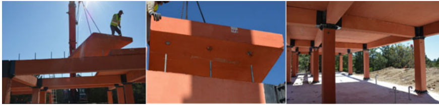
Fig. 14.9 Installation of slabs
