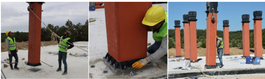
Fig. 14.7 Installation of columns
