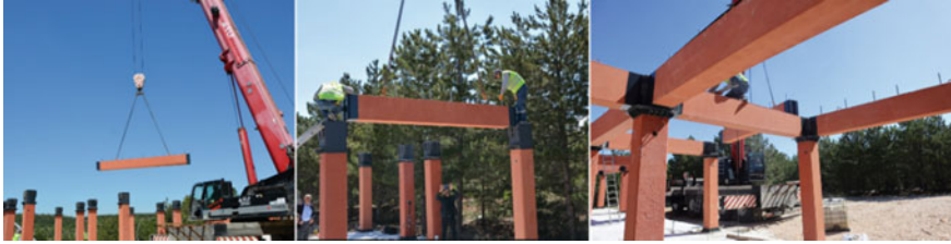
Fig. 14.8 Installation of beams
