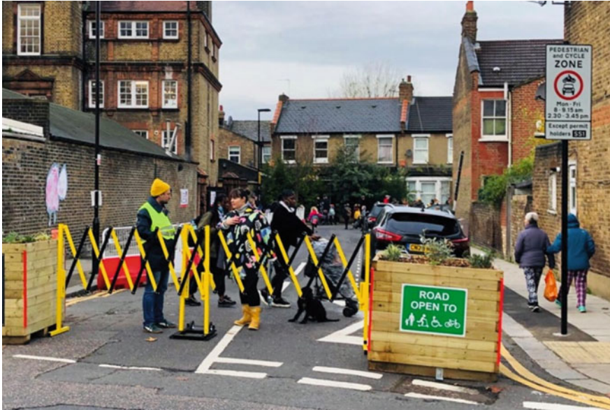
Fig. 2.4 School Street using temporary barriers in London. Source Catherine Kenyon
