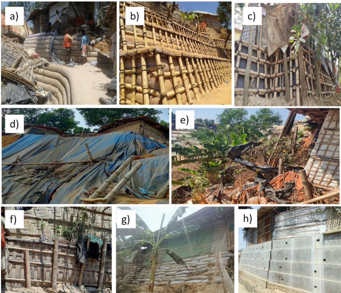
Fig. 2 Different types of structural mitigation measures exist on the slopes of the camp area (a) terrace of geotextile tubes, (b) Terrace of geotextile tubes supported by bamboo fences, (c) terrace of tin sheets
