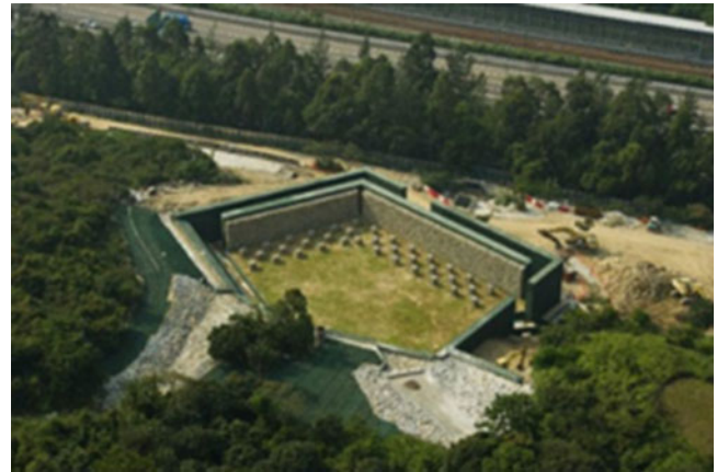
Fig. 1 Debris resisting reinforced concrete terminal barrier (modified from Ng et al. 2020a)
