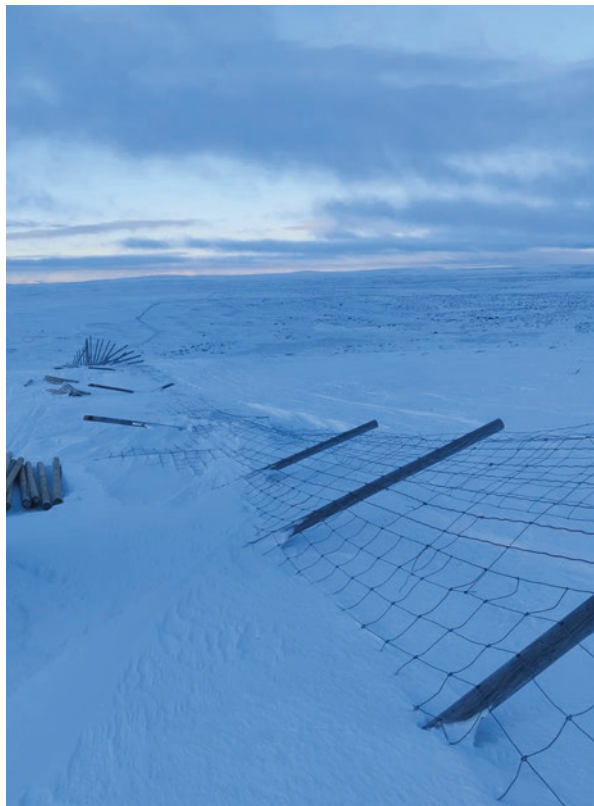
Fig. 1.3 Fallen reindeer fence between Norway and Finland in Rávdooaivi, Eanodat. The fence had fallen for several miles due to ice, snow, and strong wind combined. (Photo: Lemet Ánde Näkkäläjärvi, 2020)
