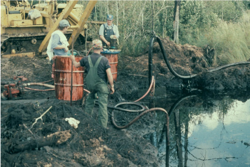
Fig. 1.2 Crude oil reached a wetland near Bemidji after the rupture of an oil pipeline. Initial efforts to remove the floating oil were conducted by the pipeline company in 1979 using pumps and other machinery (photo courtesy of Jared Trost, USGS)
