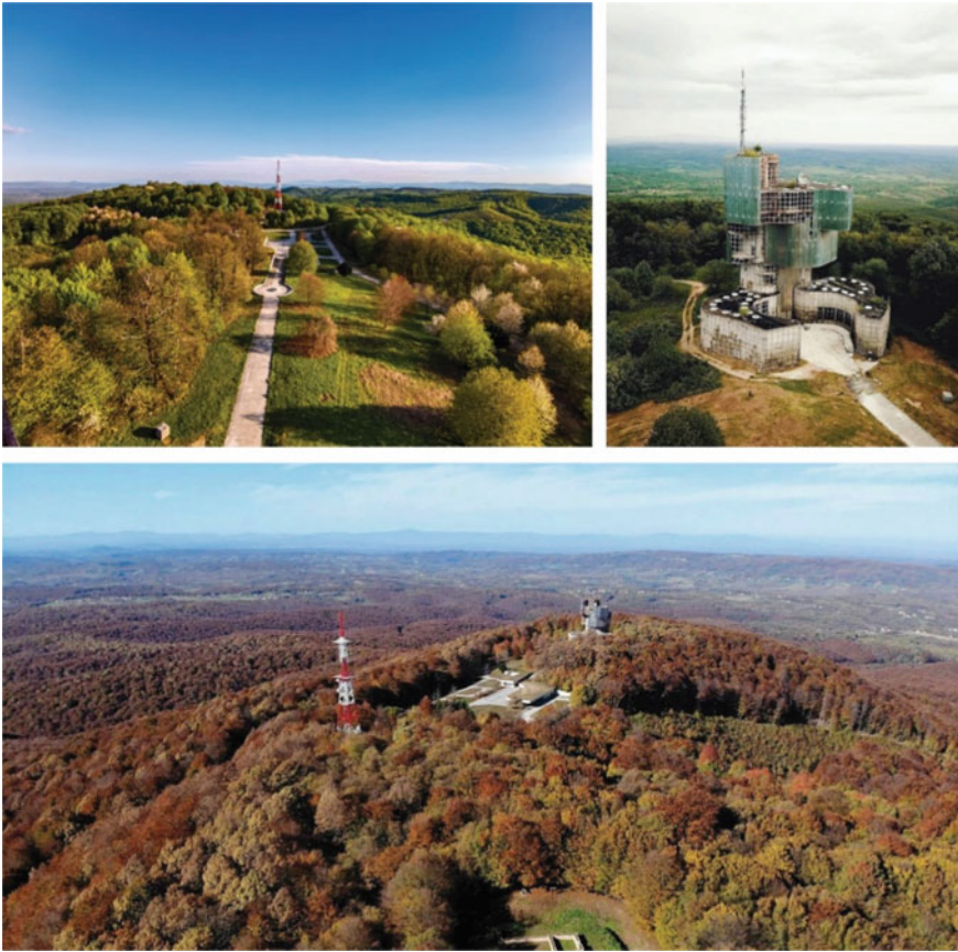
Fig. 83.2 Petrova Gora Monument—airial photography of the current state. Source Photo by Ivica Pezić, printed with permission (up left); photo by Mladen Ivanović, printed with permission (up right); photo by Alan Čapljar adopted from Planinarski izazov za ožujak (2021). https://gojzeki.com/izazov-za-ozujak/ (down)
