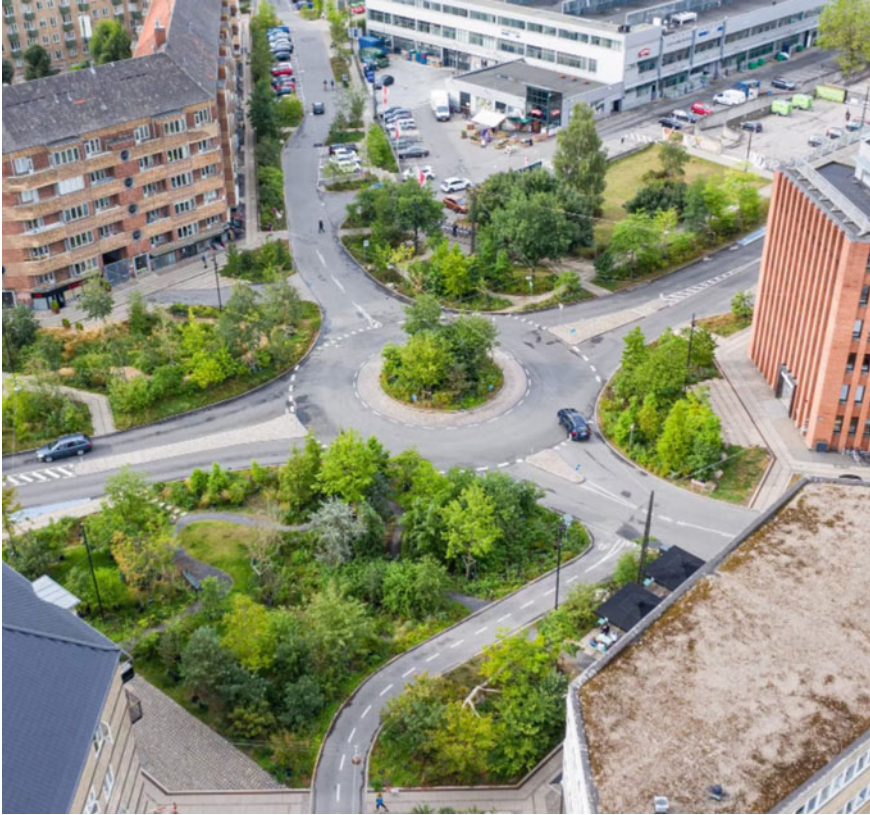
Fig. 76.1 Traffic circle Skt. Kjelds Plads and Bryggevangen road (Courtesy of SLA)
