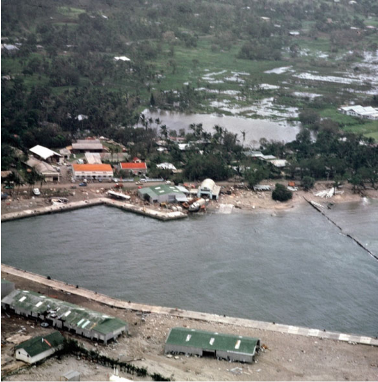
Fig. 10.5 Cyclone damage to Avatiu Port from wave and storm surge impacts (Reproduced from Blacka et al. 2013)
