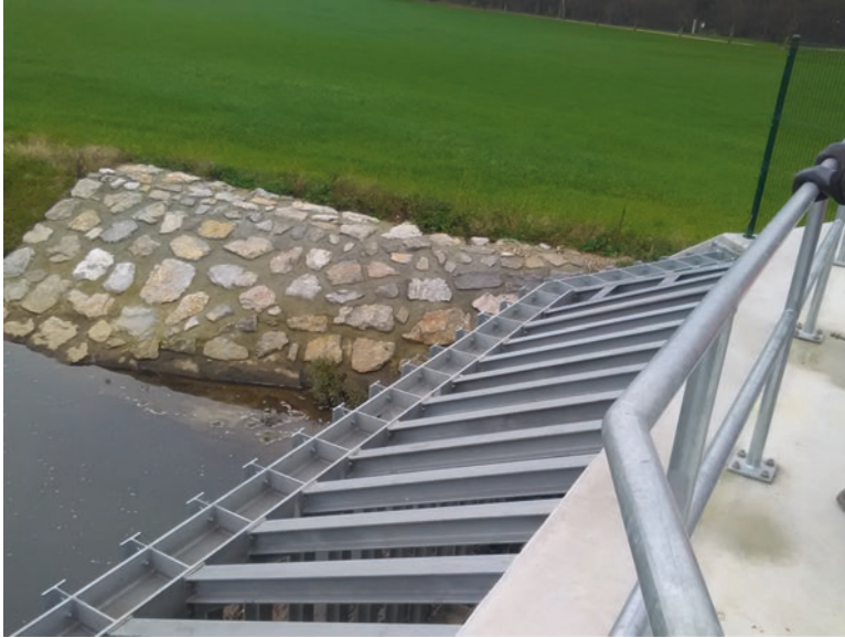
Fig. 15.5 The FreeStation was installed on the driftwood barrier at the lower end of the newly built Brdnikova reservoir
