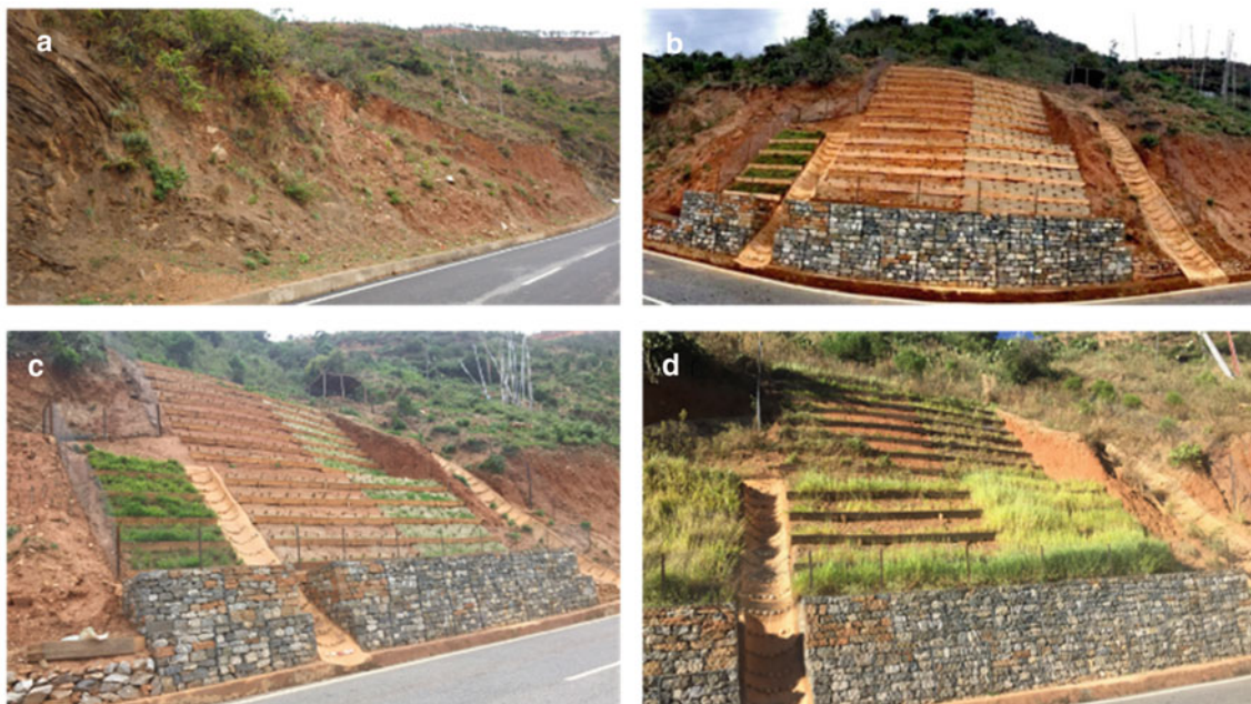
Fig. 22 Sequence of events at the site of vegetation works, Gangthangkha, Wangdue (lat 27° 29' 4.87" N, long 89° 54' 17.24" E, alt 1309 m, a slope before vegetation works on May 29, 2019, b finished
