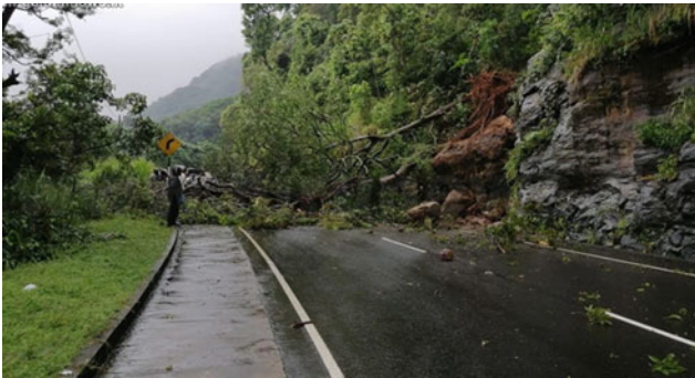
Fig. 2 Traffic disrupted (trees and rock has fallen in to the road) on to the road at 6th bend area of the Kandy-Mahiyangana “18 hairpin road”, 20th January, 2020 (Photo by Hirunews.lk 2020)
