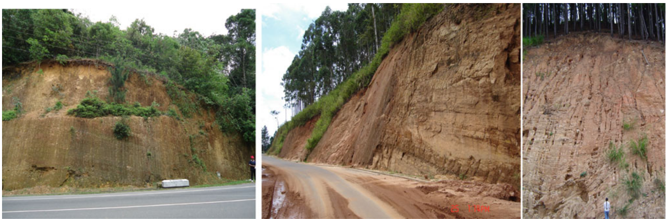
Fig. 14 Some stable landforms were also noticed during investigations. Highly to completely weathered rock surfaces consist of unsaturated soils, each having different visual and physical characteristics. Surface erosional potential is high if the weathered surface
