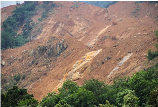
Fig. 6 Sliding surface or the point of initiation of the Aranayake landslide in Sri Lanka, 2016 Photo by Sri Lanka Red Cross (2016)
