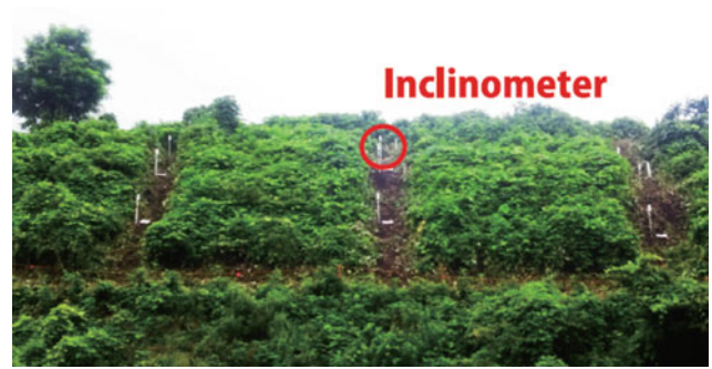
Fig. A.47 Cut slope monitoring
