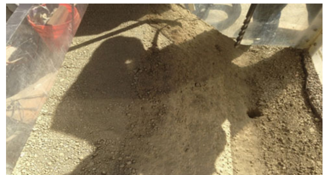
Fig. 3 Drilling in the slope to install the miniature tensiometer
