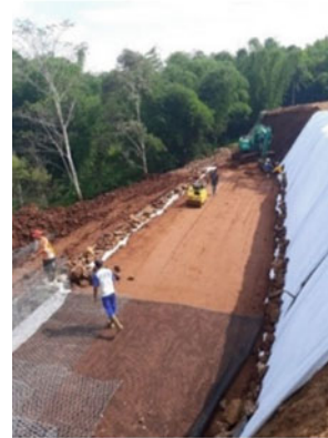
Fig. 2 Example of remediated slope with reinforced slope structure (from IGS leaflet “Geosynthetics in Slopes over Stable Foundations”)
