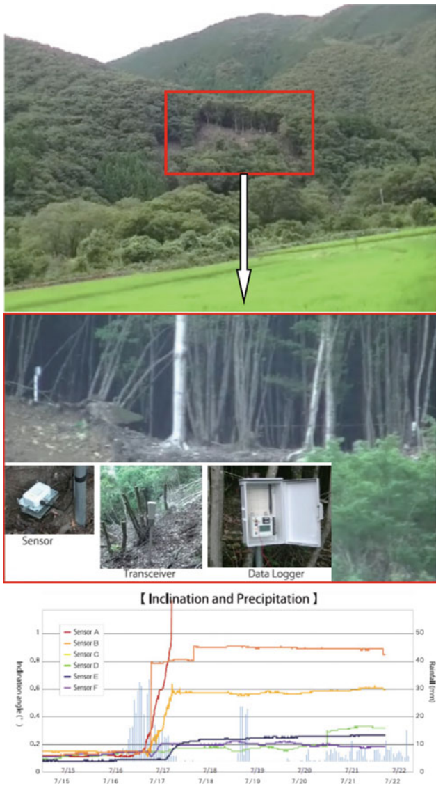
Fig. A.46 Measurement of the dynamic state of landslide using inclinometers with a wireless function
