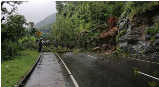
Fig. 2 Traffic disrupted (trees and rock has fallen in to the road) on to the road at 6th bend area of the Kandy-Mahiyangana “18 hairpin road”, 20th January, 2020 (Photo by Hirunews.lk 2020)
