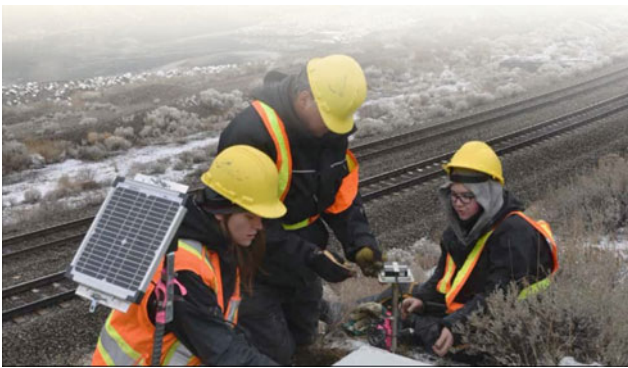
Fig. A.7 The GSC conducts geohazard studies to reduce risks to people and infrastructure, here installing equipment to monitor landslide activity above a critical railway corridor in central BC
