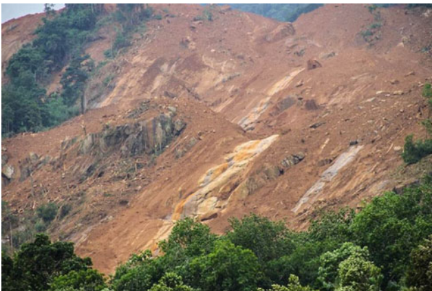
Fig. 6 Sliding surface or the point of initiation of the Aranayake landslide in Sri Lanka, 2016 Photo by Sri Lanka Red Cross (2016)
