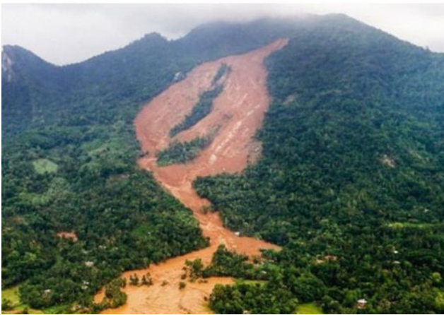
Fig. 5 Aranayake landslide in Sri Lanka is now thought to have killed about 122 people. The landslide was triggered by an exceptional rainfall associated with a slow-moving tropical cyclone, 2016. Photo by Sri Lanka Red Cross
