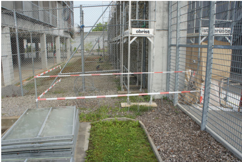
Fig. 5.1 Scaffolds installed on the prison grounds (Source Photo by a prisoner)
