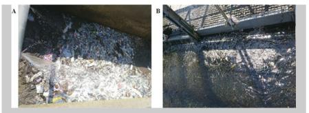
**Image 2.1** Evidence of debris in the **a** dissolved air flotation tank and **b** effluent of a Cape Town WWTP (Chitaka, 2020)
