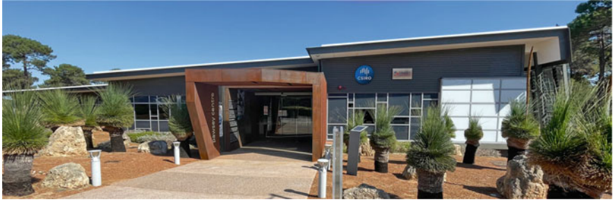
Fig. 37.15 Pawsey Supercomputer Centre at Kensington, Western Australia. Credit: Pawsey Supercomputing Centre
