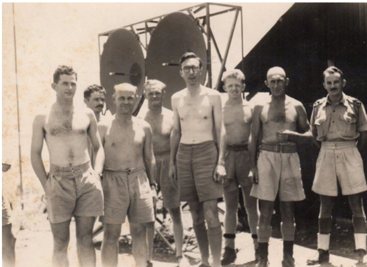
Fig. 9.4 Coastal Defence Number 1 (A 272 MkI), a coast watching radar set (Army). Two antennas used in order to improve bearing determination. This radar could function as a coast artillery directing set providing precise azimuth and range determinations of ships up to 45 miles. Location likely Northern Territory. Pawsey is the tall man fourth from the right. Credit: Joe and Lenore Pawsey Family Collection
