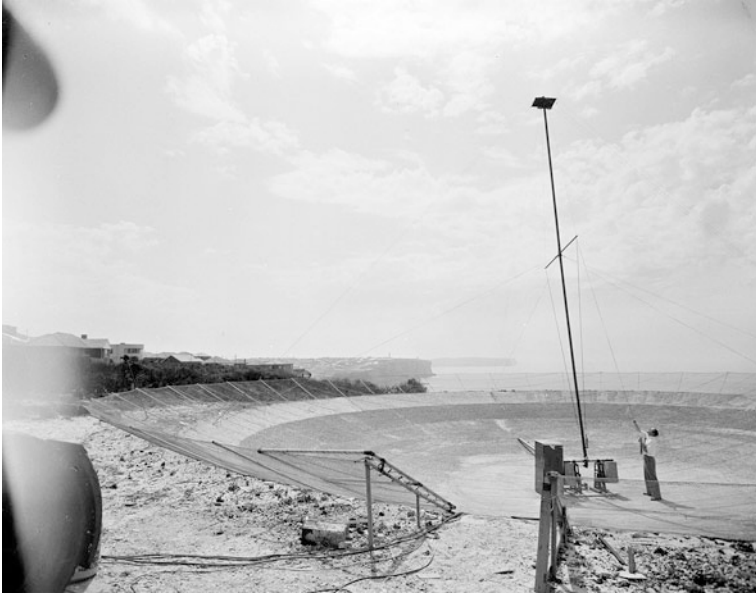
Fig. 23.4 The newer more accurate 80-foot dish at Dover Heights. Dick McGee adjusts the mast. View to the north towards North Head and the Sydney Harbour entrance. Credit: CSIRO Radio Astronomy Image Archive B3150-1
