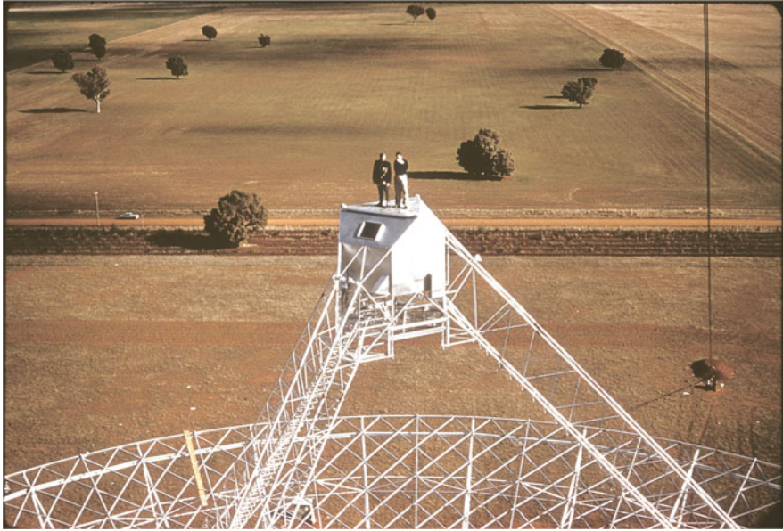
Fig. 32.2 Harry Minnett (left) and Dennis Gill in June 1961 on top of the Parkes telescope aerial cabin, as photographed by George Day from the erection crane. Credit: CSIRO Radio Astronomy Image Archive JP32-2
