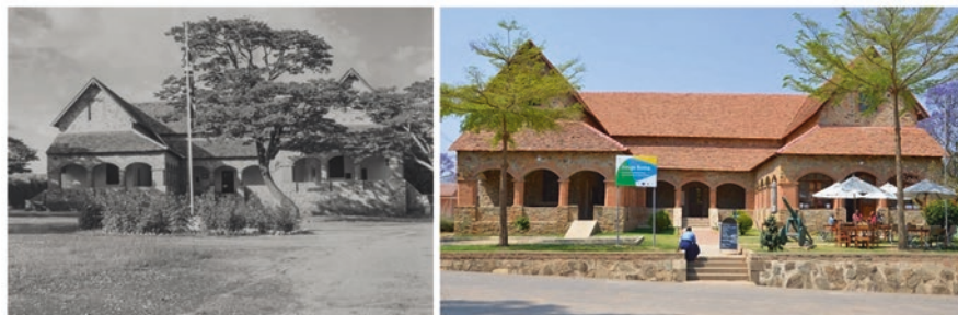
Fig. 11.1 Iringa Boma during British administration (Troll, 1934, left), after restoration in 2016 (right). (Note. Photograph (right) by fahari yetu Tanzania. Printed with permission)
