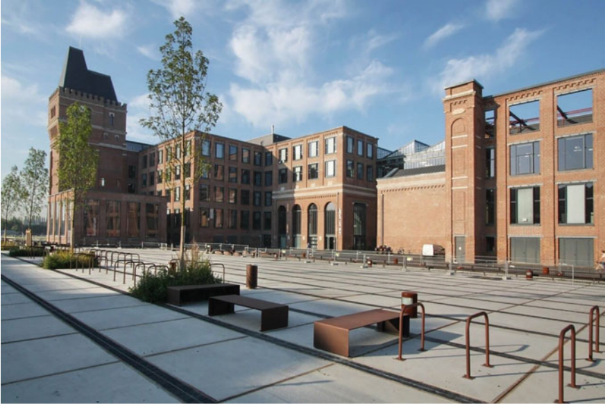
Fig. 3.2 EuraTechnologies Campus, Lille (FR). Transformation of a former spinning mill into a start-up incubator and accelerator. B + A Architectes, 2009 (photo: Stefan83~fwiki, 2018)
