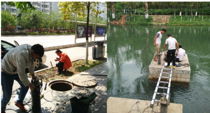
Fig. 5.11 Implementation of monitoring equipment
