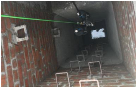
Fig. 7.13 Inserting the prototype II into the sewer. (JT Elektronik)
