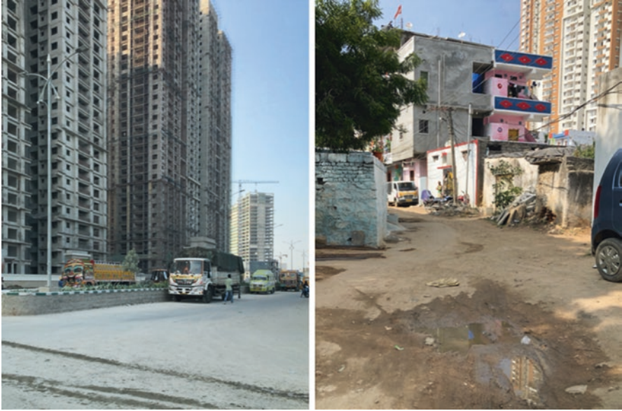
Fig. 5.1 High-rise gated developments (left) and the adjacent neighbourhood (right) in Nanakramguda. (Photos by authors)
