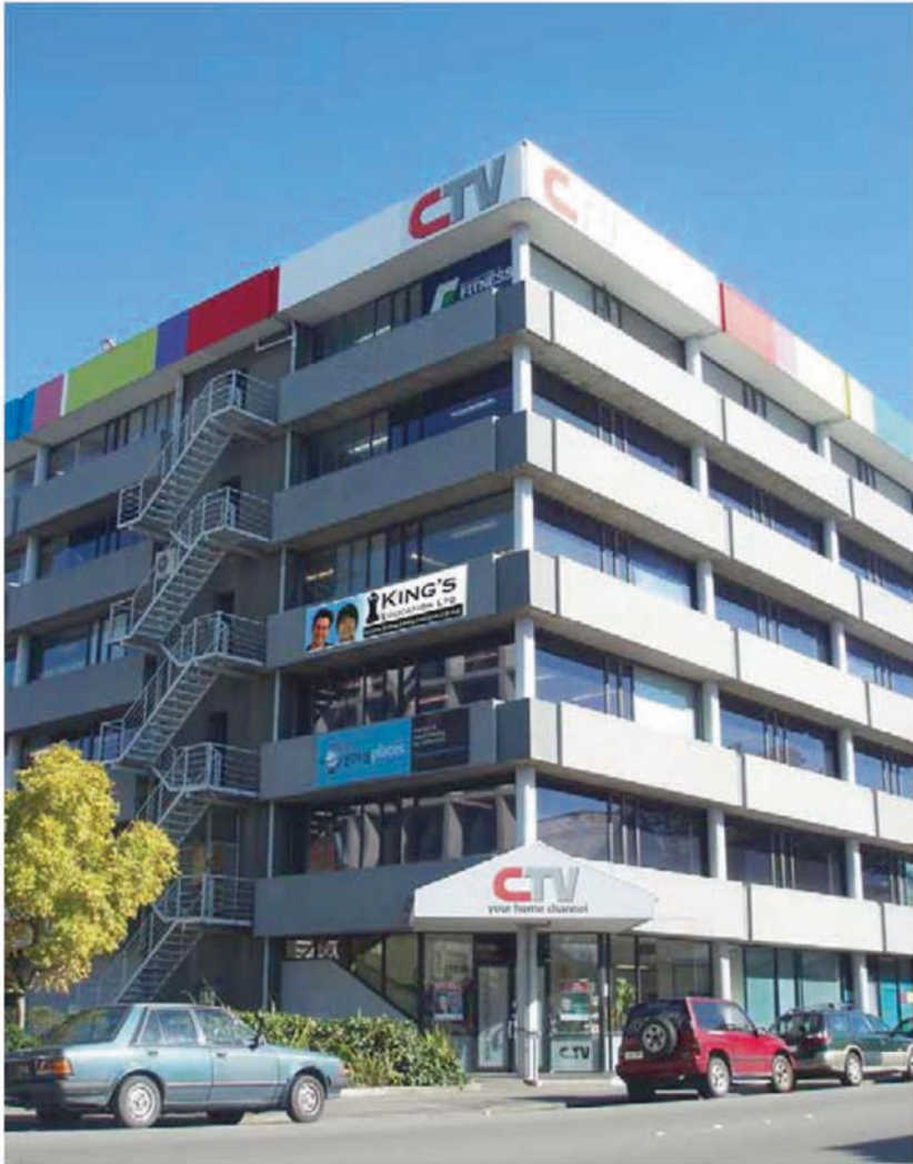
Illustration 4.1 CTV Building Christchurch prior to its collapse on 22 February 2011. (Source: Royal Commission Vol. 6, p. 3)
