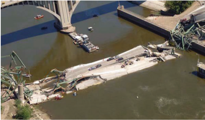
Illustration 3.1 Collapsed I-35W Bridge center section. (Source: NTSB Report, p. 19)
