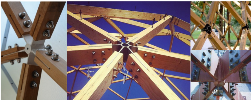
Fig. 1. Splice node-connection “POLO-1” [9, 10].
