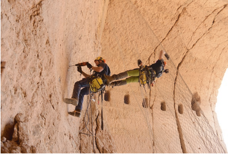
Photo 10 Western Buddha niche, September 2017: Prestabilisation measures on Western Buddha rear face, former head area (BRR-team Klaus Vogt und Stephan Hardt). (© Bert Praxenthaler)
