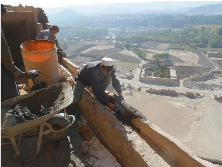
Photo 9 Western Buddha, October 2013: Repair of the water channels. (© Bert Praxenthaler)
