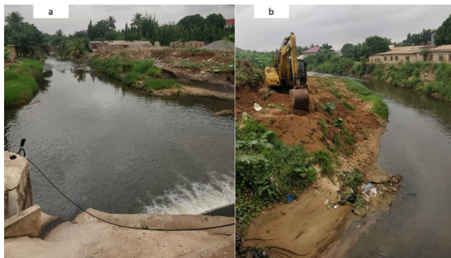
Fig. 2 (a) Location of residential buildings near open drainage and (b) excavation and disposition of dredged materials to drainage banks, which lead to rapid re-siltation and increases flood risk in Accra
