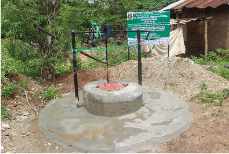
Fig. 8 A dug well for improved economic activities by the intervention
