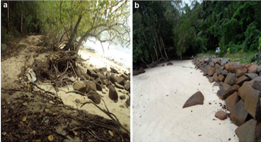
Fig. 4 Severe erosion at Anse Marie-Louise on Praslin Island highlighting coastal erosion (a) and the construction of rock armoring (b) to mitigate the impacts of coastal erosion (MEECC 2019)
