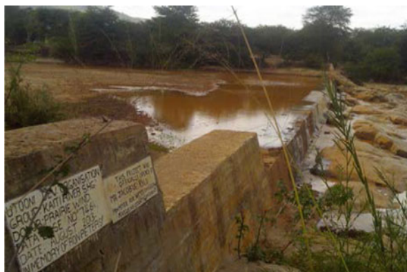
Fig. 13 A sand storage dam construction in Makueni County during the dry season (Photo taken by Mary)
