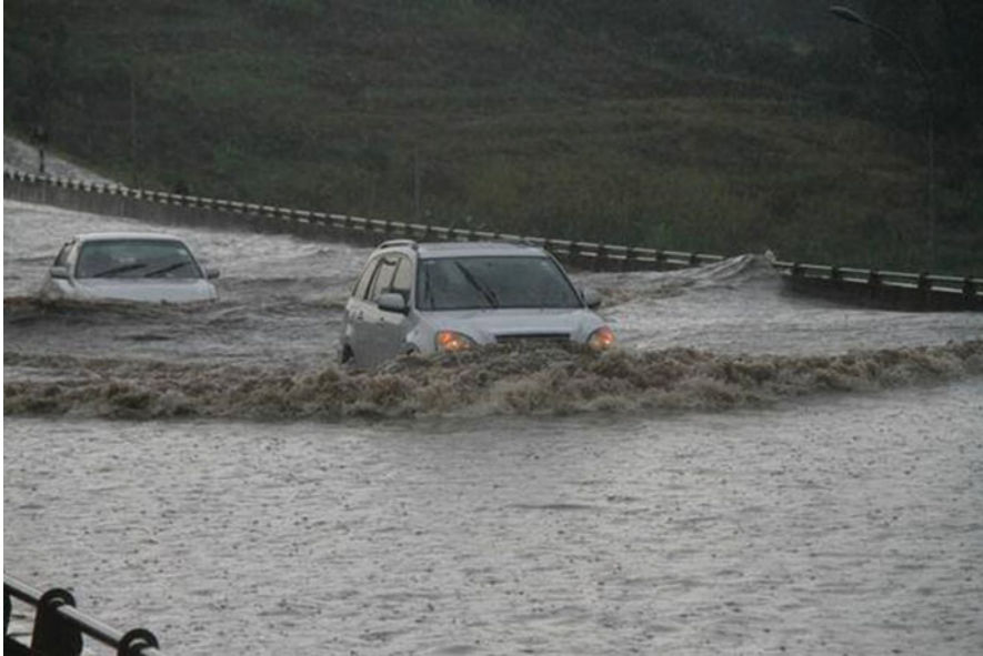
Fig. 8 A flooded Thika superhighway after a downpour
