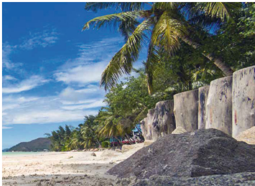
Fig. 5 Timber piling for coastal protection on Praslin Island (World Bank and MEECC 2019)
