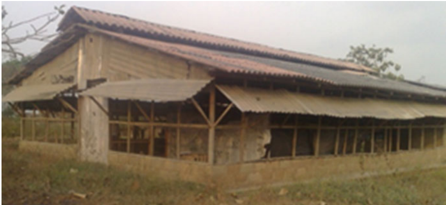
Fig. 3 Low-walled broiler housing units
