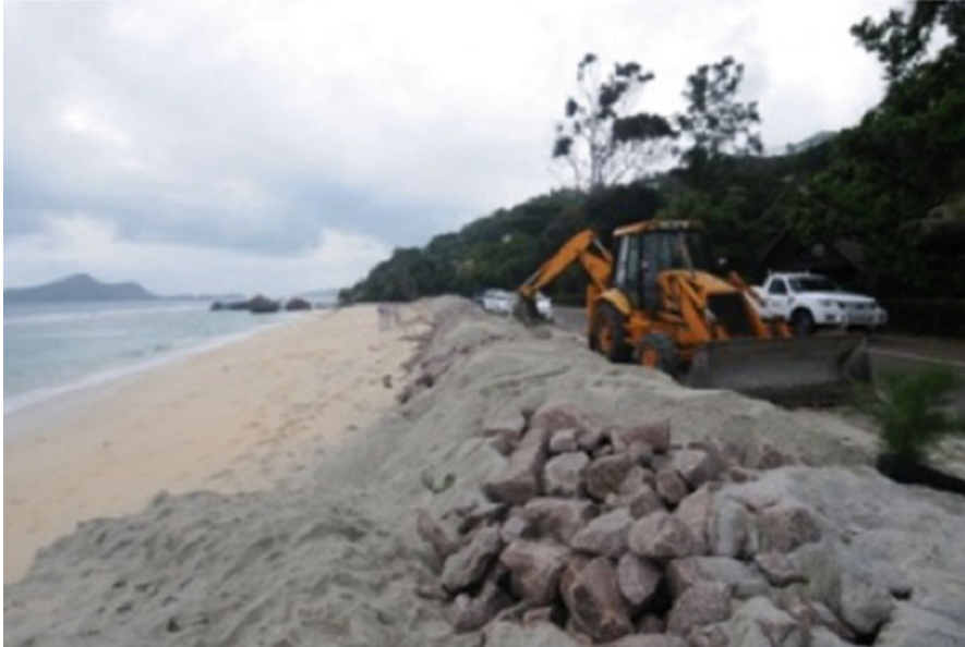
Fig. 6 Beach nourishment project at the North East Point beach, Mahé Island (MEECC 2019)
