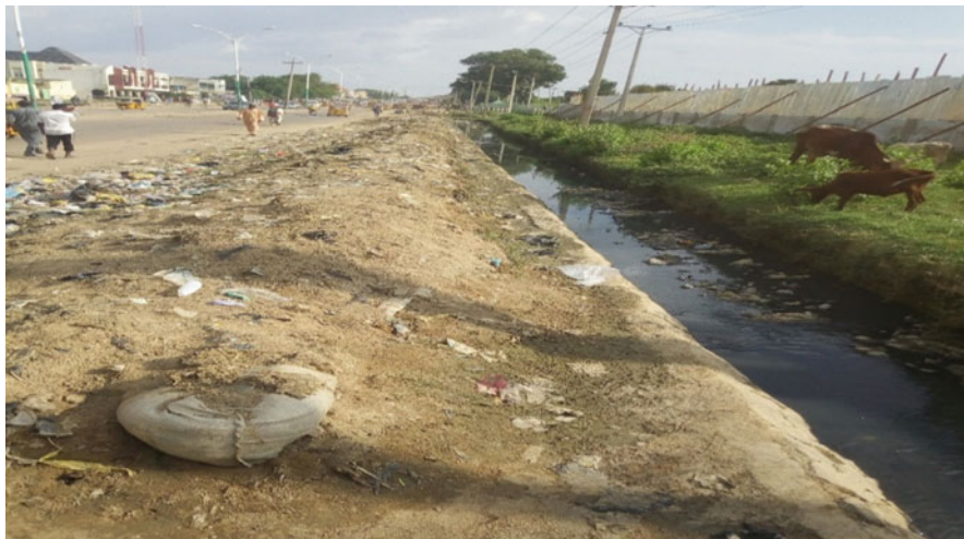
Fig. 11 De-siltation of drainages to improve free flow of storm water, but not properly evacuated which have tendency of finding its way back into the drainage
