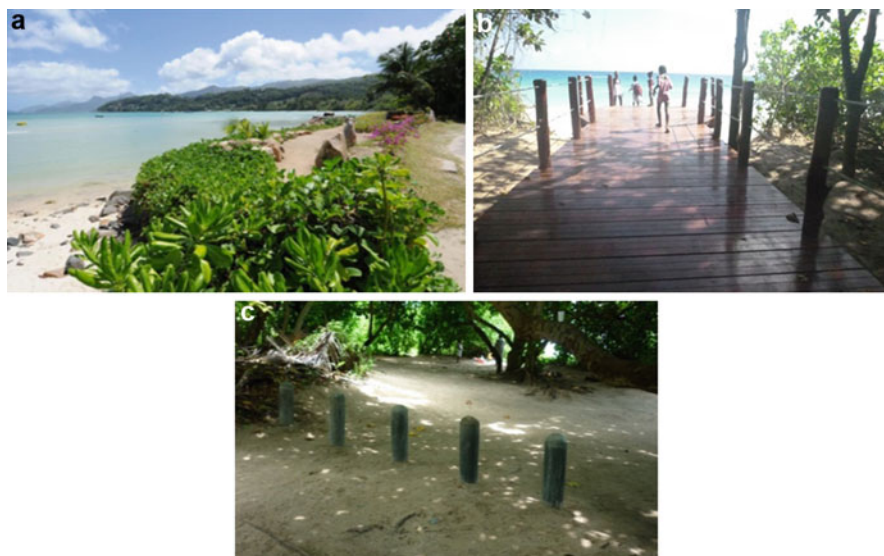
Fig. 7 Re-vegetation at Anse à La Mouche (a), constructed boardwalk at Grand Anse (b) and bollards (c) to protect dune-land from vehicles at Anse Royale (MEECC 2019)
