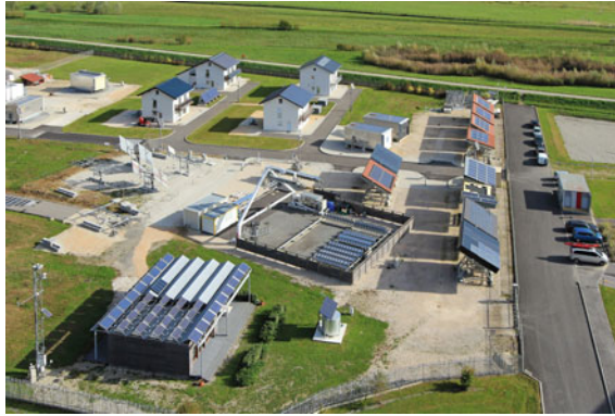
Fig. 12 The houses and PV packs considered in the microgrid
