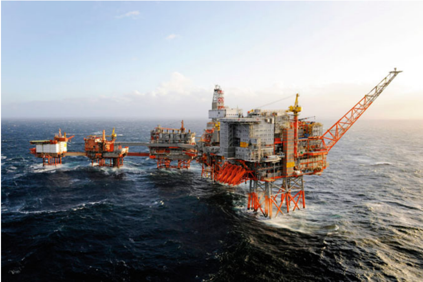
Fig. 5.6 A platform rig in operation. (AkerBP)
