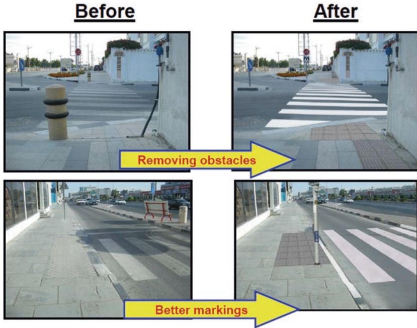
Fig. 5.1 Proposed changes as stipulated in the RTA’s comprehensive Strategy for People of Determination; examples from Jumeirah Beach Road, Dubai
