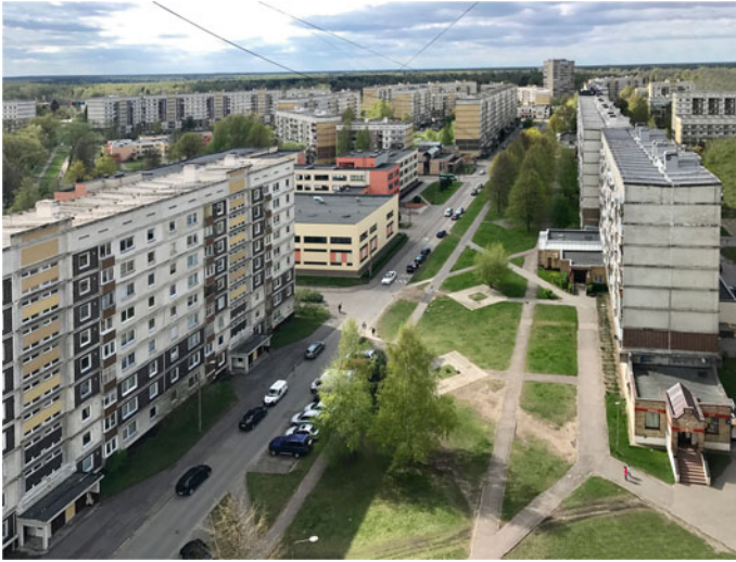
Fig. 8.2 Main inner street with pedestrian priority and services in mikrorayon Zolitūde I (arch. Berķe et al.). Source Sandra Treija
