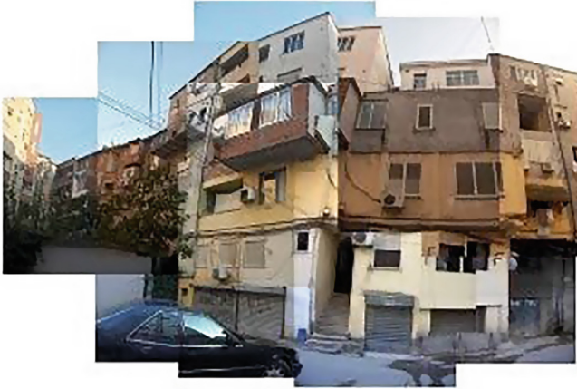
Fig. 4. Abusively added volume in Tirana
