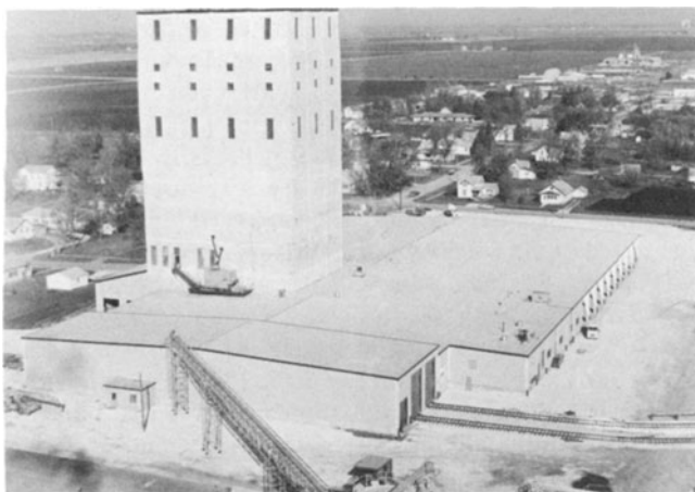
Fig. 4. Overall view of modern feed mill, showing mill tower and rail and truck receiving and shipping connections. (Boone Valley Co-op Processing Association, Eagle Grove, Iowa)
