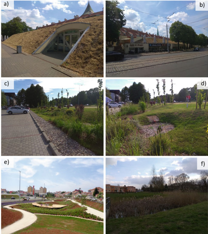
Fig. 2 Examples of NBS in urban areas: (a) green facade and (b) green roof in Riga, Latvia, (c) bioretention basin and (d) infiltration trench in Riga, Latvia, (e) detention basin in Pula, Croatia, and (f) wetland in Ghent, Belgium
