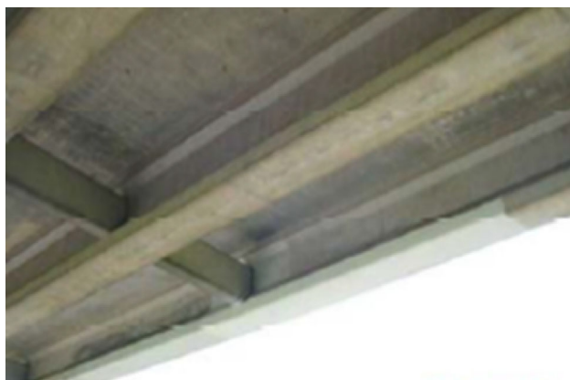
Fig. 1 CFRP strengthened concrete bridge girder
