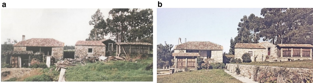
Fig. 5 Casa da Eira: a 2 nd phase before intervention; b after intervention
