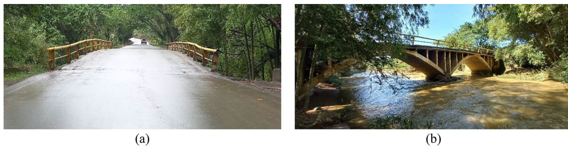
Fig. 5 The Río Claro Bridge: a Road view b Isometric view
