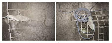
(b) Step 2 Shotcreting and burring stress meter (c) Step 3 Leading wires and connectors
