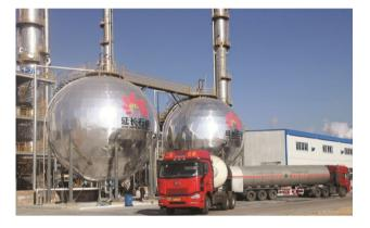
Fig. 3 50,000 tpa  $\mathrm{CO}_2$  capture facility in Yulin Coal-Chemical Company
