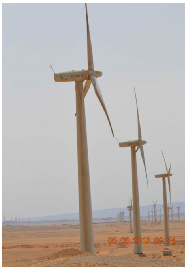
Fig. 1 Nordex wind turbine towers at the Zafarana wind farm
