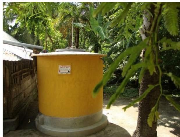
Fig. 4 Rainwater harvesting tank (4,500 l) for reducing drinking water risks, Morrelganj, Bangladesh. Photograph by S. Samaddar, August 2012
