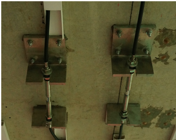
Fig. 12 Realistic diagram of sensors' installation.
