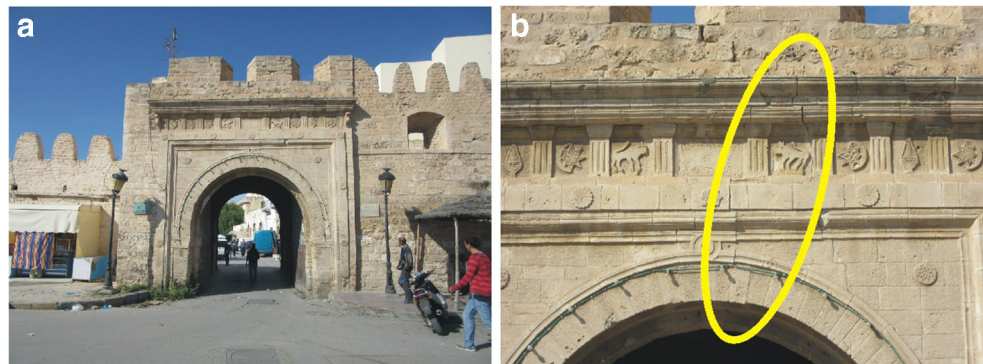
Fig. 8 Slightly damaged arch of the southern gate to the medina , Monastir. a Monastir, medina , southern gate. #6193. b Left part of gate subsided. Displacement extends up to the ledge, going around all masonry blocks (circle). #6194. I = VII. 35^{\circ} 46' 22'' N, 10^{\circ} 49' 50'' E
