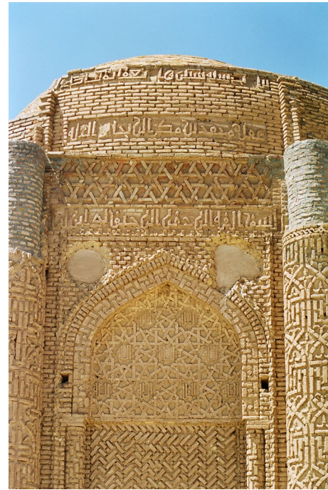
Fig. 16 Frieze: a pattern of nested hexagons and hexagonal stars with a (partly obscured) layer group p622 ; a cut-out of a 2D pattern. Tympanum below: A complex hexagonal pattern (layer group p622 ) with ‘Allah’ written in the 12-fold star-shaped recesses. Intervening wall: a brick layer course cm with plugs between bricks. N panel of the E tower
