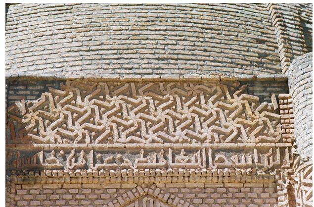
Fig. 17 A p6 pattern of shaped bricks in the frieze of the NNE panel; W tower. A simple pattern with one type of recessed fields, positioned on threefold rotation axes
