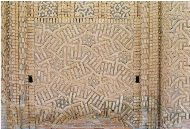
Fig. 21 WNW panel of the W tower. A p6mm tile scheme altered into the p6 pattern by presence of swastikas, which became reduced to blocks consisting of parallel bricks by a loss of plaster cross-arms during weathering. The apparent symmetry today is p2
