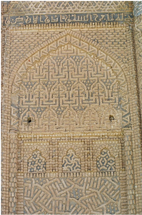
Fig. 27 The WNW panel of the W tower. Tympanum: a cm pattern of complex upward pointing elements and dotted infill. Note similarity of design to the cm buttress pattern in Figs. 25 and 26. Niches: two types of p6 patterns and the p4gm pattern of ‘pointed parentheses’
