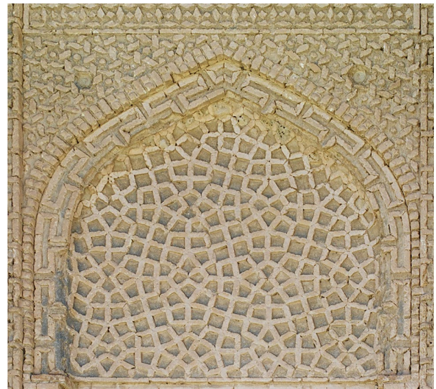
Fig. 13 The complex p4gm rib pattern of squares, lozenges, triangles, and pentagons, with superimposed dual lines. Surmounted by a diaper p6 pattern and a linear p2mm pattern. The NNW tympanum panel of the W tower
