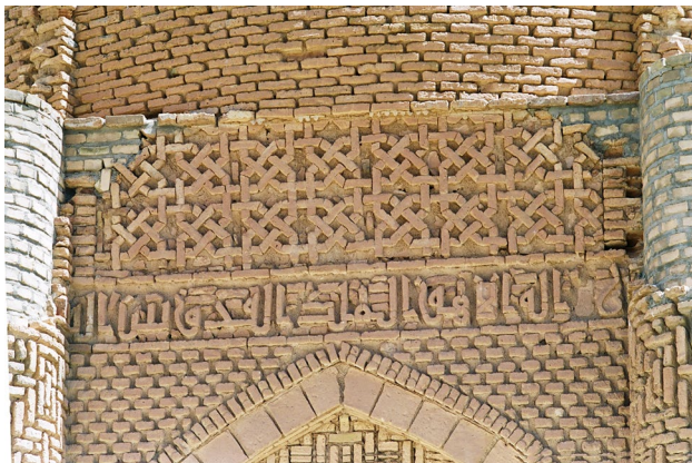
Fig. 12 A pattern of interwoven ribs with a layer group p422 . E tower. This patterning of conspicuous fourfold rosettes actually is a pattern of overlapping octagons, which are present as 4+4 octagons for each central octagon. See also Fig. S14, the top frieze
