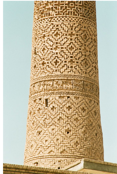
Fig. 28 The bottom portion of the Damghan minaret is conical and the (possibly intended) p4mm flat-brick pattern becomes split and modified in its lower half. At the top of this portion, a repetition of nine ‘standing’ bricks and 14 lying bricks results in the cmm pattern with a separation of horizontal zig-zag strips. In the conical bottom portions, we observe a growing misfit of strips. In the cylindrical top portion, a 16 \times 16 brick pattern creates large squares, spanning seven bricks, and is modulated by empty squares and braided fragments; plane-group symmetry p4mm . Graphic illustration of this pattern is in Makovicky (1989), (his Fig. 23)
