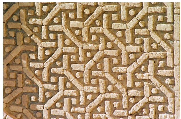
Fig. 10 An expressive p4gm panel with a double-Y (double-fork) pattern in the tympanum of the W tower. Twin forks are positioned on twofold axes and intersection of reflection planes, i.e., in 2mm positions. The loose square configurations are situated on fourfold axes. SSE panel of the W tower
