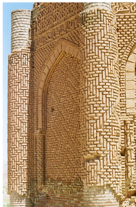
Fig. 5 Two members of the homologous series formed by a square-based p4mm pattern, with 7 and 11 tiers counted along the vertical diagonal of the unit square, covering two separate buttresses. A framed p4mm pattern of squares and crosses covers the intervening flat panel. Buttresses flanking the S panel of the E tower
