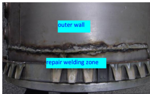
Fig. 4 The repair welding zone of the outer wall
